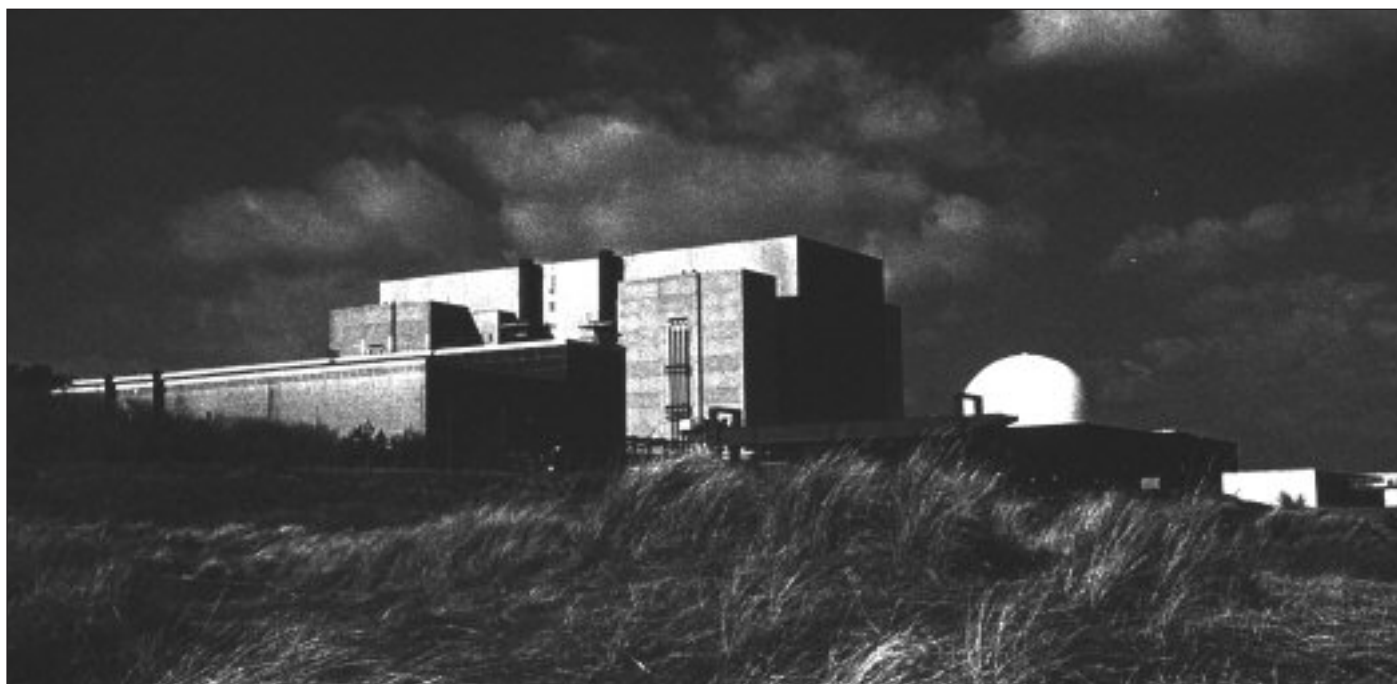
Sizewell nuclear power station
